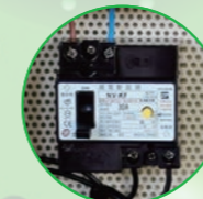
LEAKAGE CIRCUIT BREAKER
